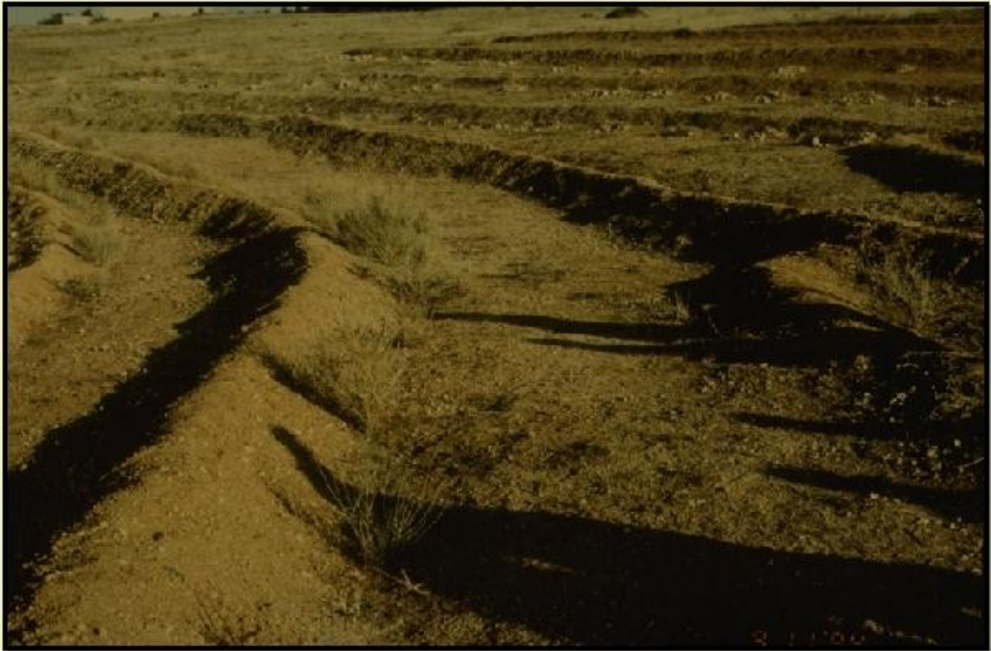
Contour bunds after construction and before planting; Photo: Prinz
