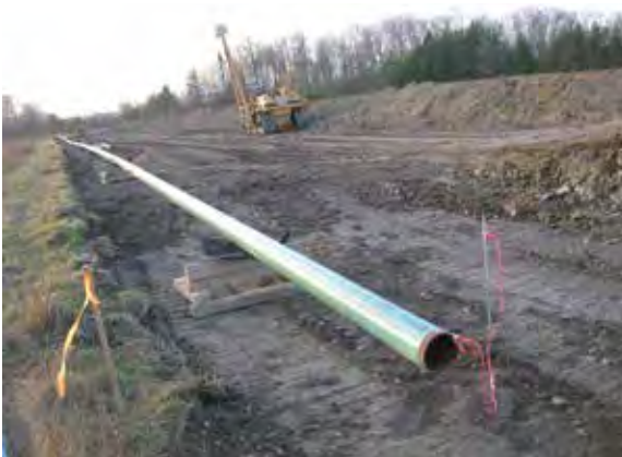
Figure 22.7. Proper pipeline construction: Left: fertile topsoil is first removed and separately stockpiled from the subsoil. Right: After installation the topsoil is restored over subsoil. Photos by Bob Schindelbeck.
