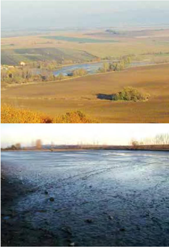
Figure 14.10. Top: A sediment control basin in a Central European landscape where conventional tillage is widely used. Bottom: Sediment regularly fills the basin and needs to be dredged.
