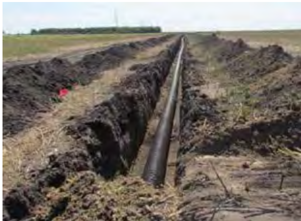
Figure 17.14. Left: clay (tile) pipes were commonly used to improve drainage. Painting by L.A. Ring. Right: Flexible corrugated PVC drains allow for rapid and durable installation. Photo by Morin Farm Drainage.
