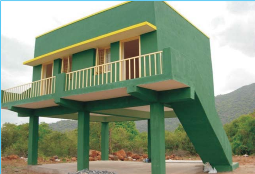
Anti-poaching shed constructed at Sathyamangalam division under Tamil Nadu Biodiversity Conservation and Greening Project
