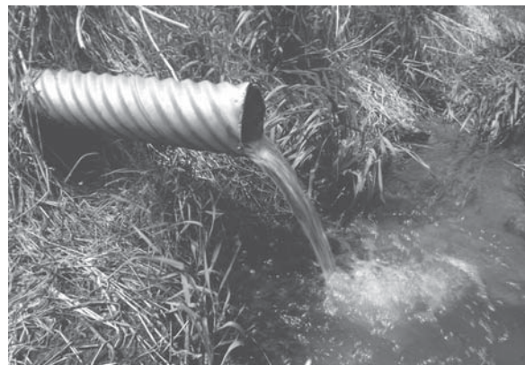
Figure 12-30 Illustration of a drainage tile transporting soil water containing NO 3 - from a field to nearby surface water. (USGS, 2010, Circ. 1350.)
