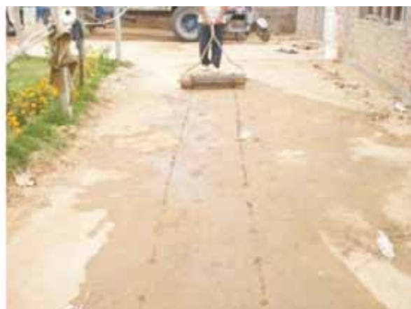
Marking done by the marking roller
