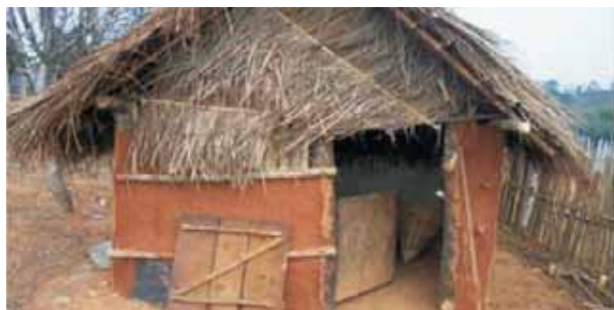
Clayed bamboo wall structure for storing ginger
