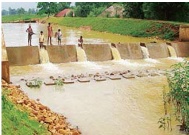
Check Dam in Jharkhand
