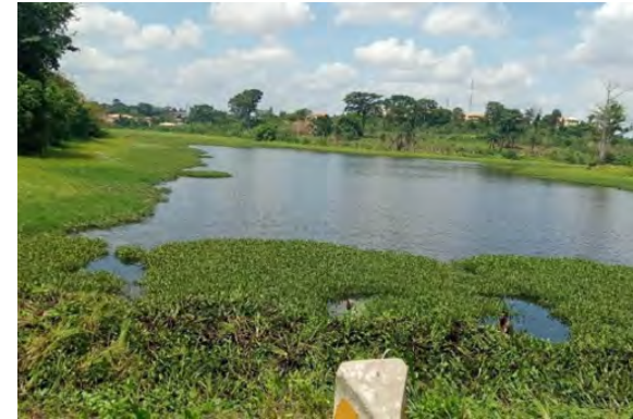
Fig. 26. Top photo: High siltation and growth of aquatic weeds on Awba Dam Reservoir, Nigeria
