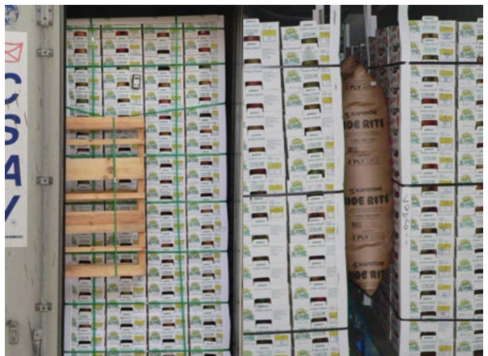
Use of blocking and air bags to stabilize loads in containers and trailers. Note the temperature recorder in the picture on the left.
